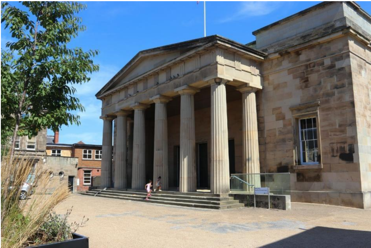
Fig 11: Front of Shirehall building
